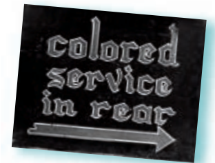
Segregation sign from the turn of the century
